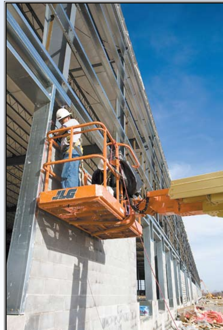
Workers erect Mericle’s new speculative building in Humboldt North.
