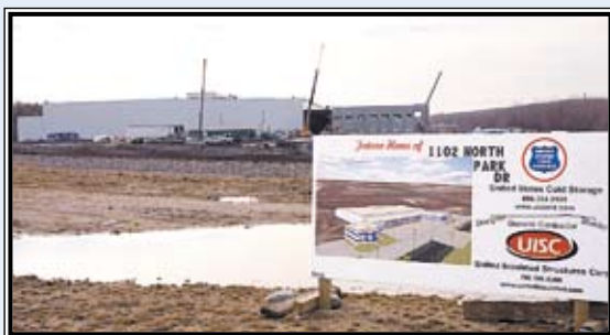
U.S. Cold Storage under construction in Humboldt North.
