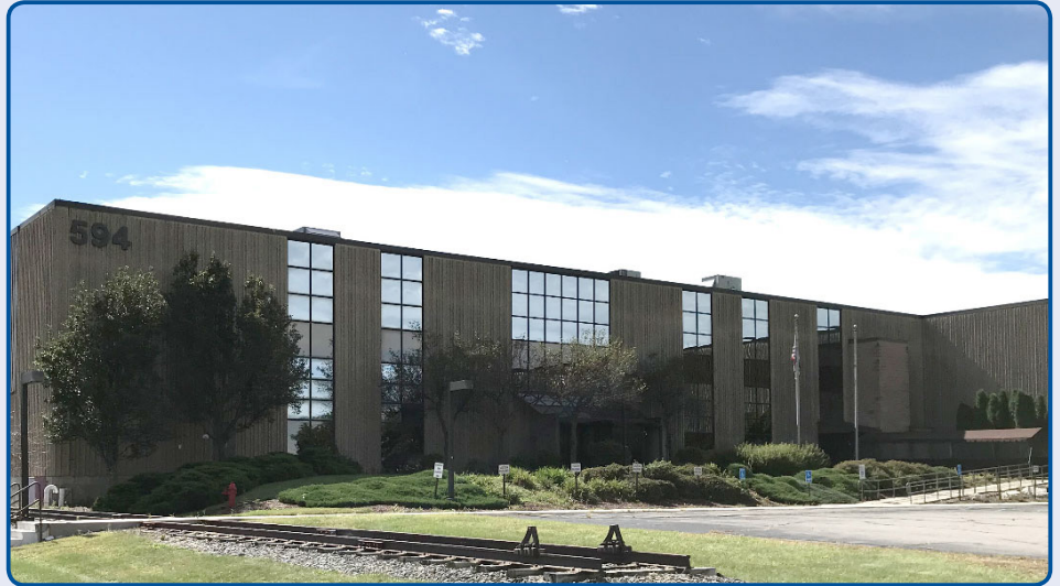
Endurance Realty Group, LLC, purchased a 242,960 square-foot Class B manufacturing and distribution facility in Humboldt Industrial Park.
