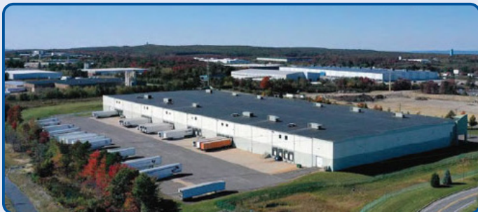
The facility at 490 Forest Road offers suites ranging from 120,000 square-feet up to 240,000 square-feet.
