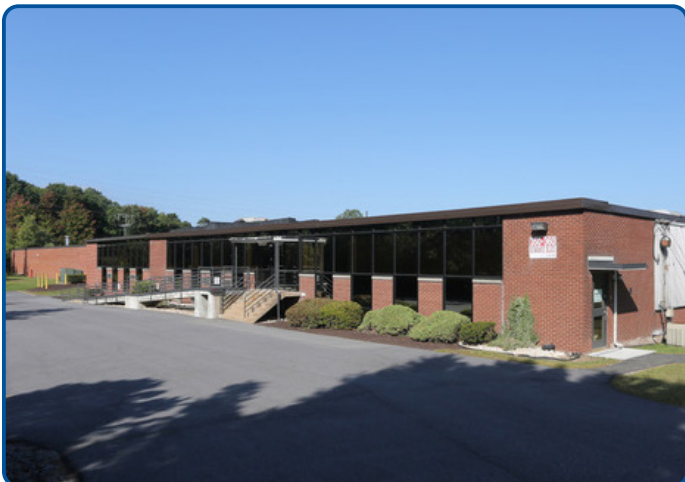
Muzo expanded its manufacturing and moved its global headquarters to this 74,000 square-foot facility in the Valmont Industrial Park in West Hazleton.
