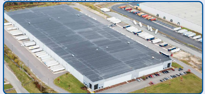
At 68 Green Mountain Road, 200,130 square feet of this 400,260 square-foot facility is available for lease.
